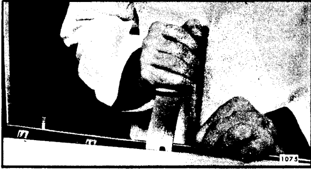
Fig. 6-118-Weatherstrip Removing Tool
